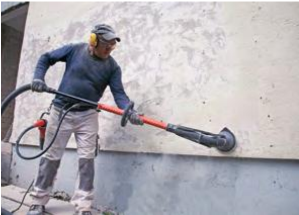
Removing old plaster and paints
