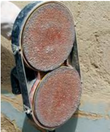
Removing old plasters
