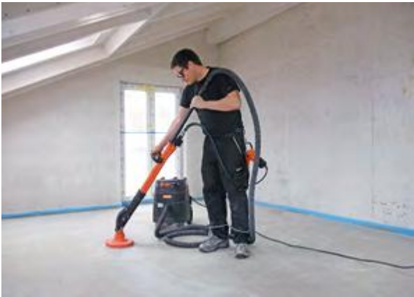
Grinding screeds
