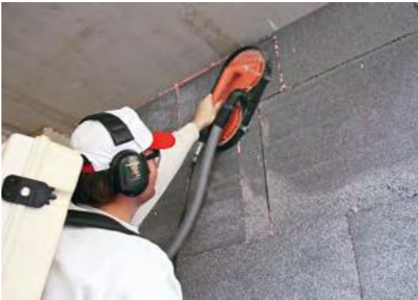
Grinding EIFS and ETICS boards
