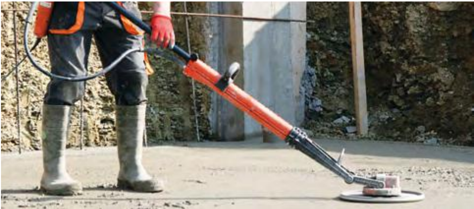
Levelling fresh concrete
