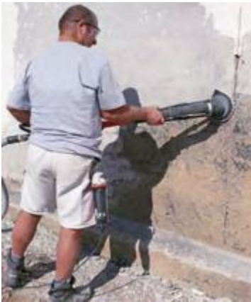
Grinding bitumen coating with PCD grinding disc
